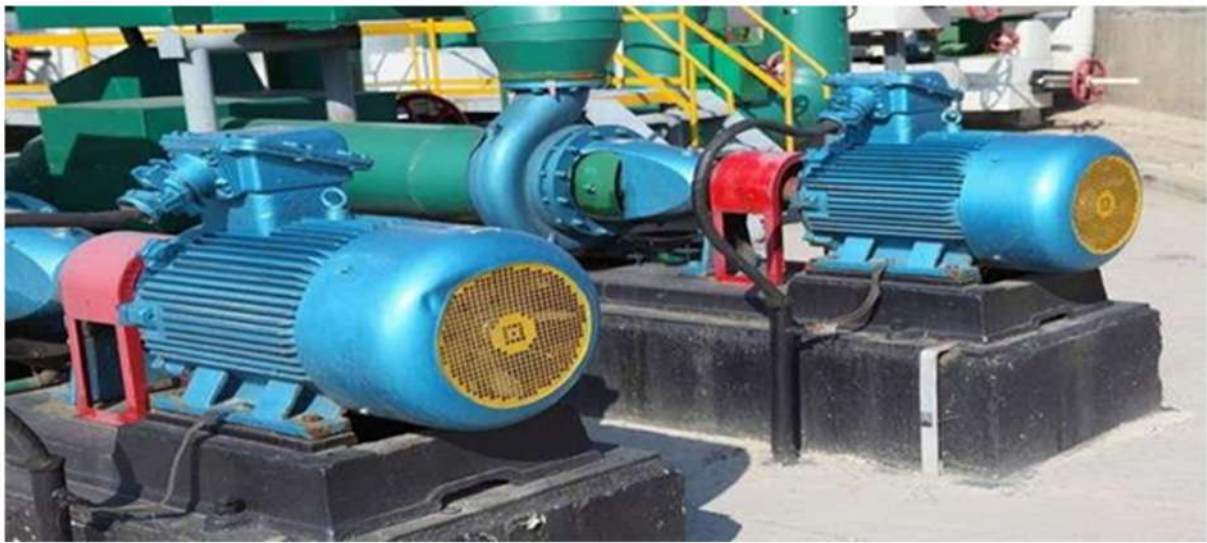
Pump House with IE3 Motor at SECL
