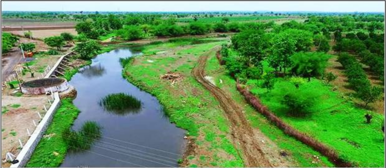
Mine water supply for irrigation from Saoner to Borgaon, WCL
