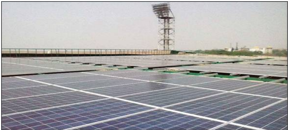
NLCIL: Solar Power Panel in Ramanathapuram District
